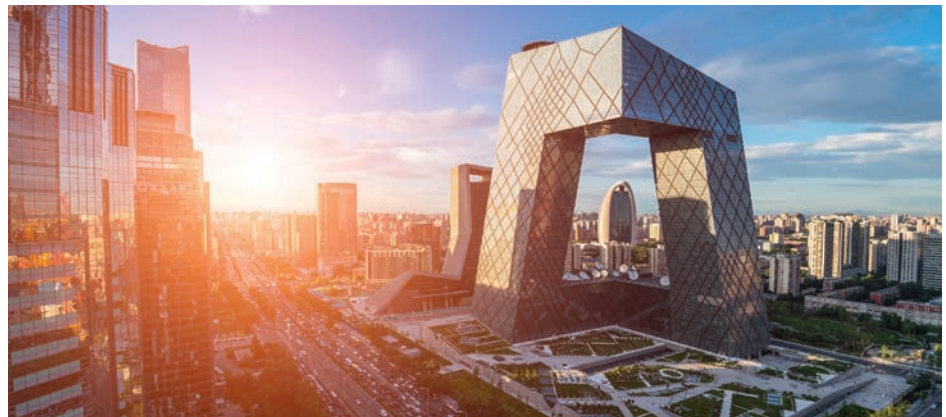
The Beijing central business district is the primary area of finance, media, and business services in Beijing, China.
