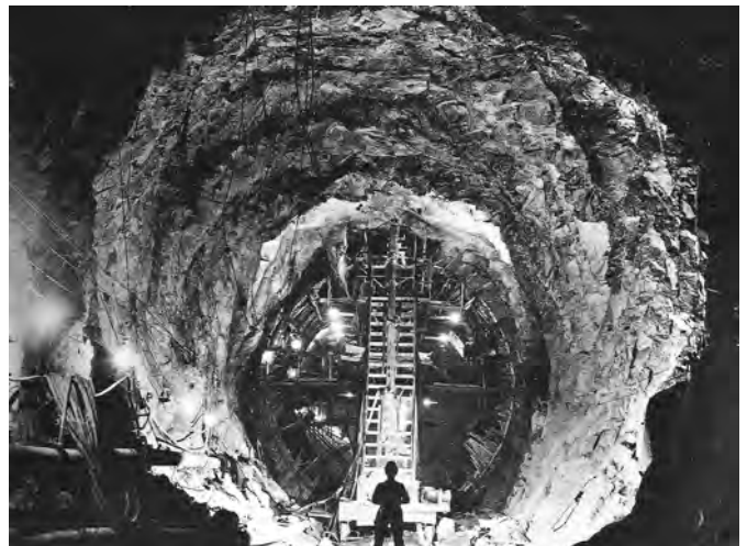
Tumut 2 tailwater tunnel during construction. Image courtesy SMEC collection.
