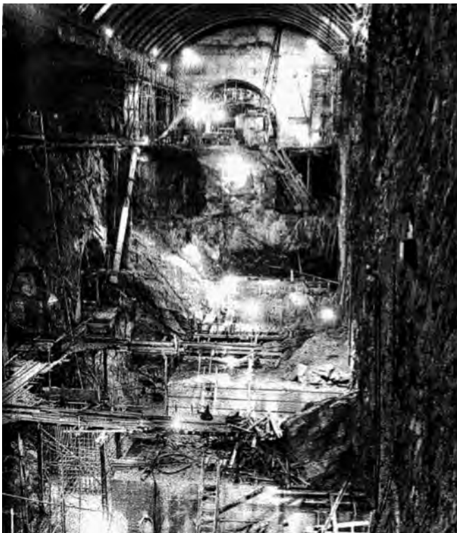
Tumut 2 power station cavern under construction. Image courtesy SMEC collection.
