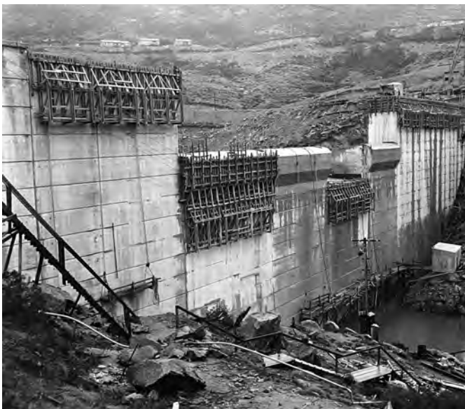
Guthega Dam under construction – image taken in 1954. Image courtesy SMEC collection.
