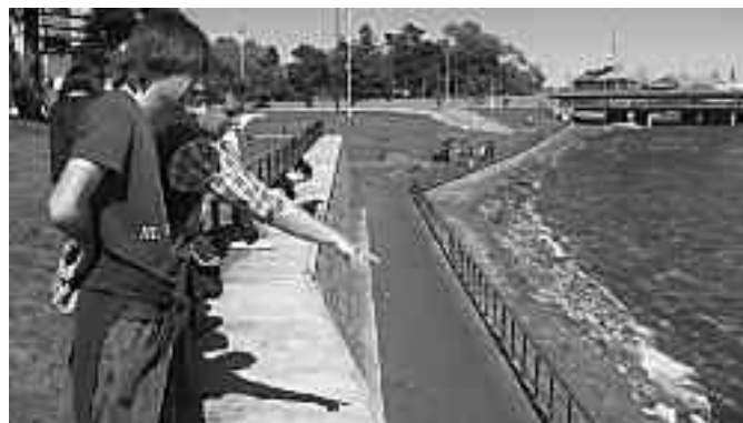
Local teachers and mentors observing flood damage along the Tapalque River, Olavarría, Argentina, site of the ITFI. Image courtesy Sabine Seidl.
